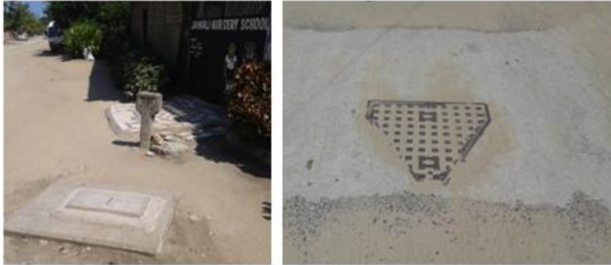
Figure 6.3: Sewerage pipe inspection chamber along street number 8 road
