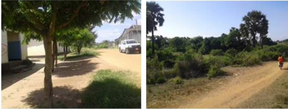
Figure 6.1: Trees located close to the project roads which may have to be uprooted
