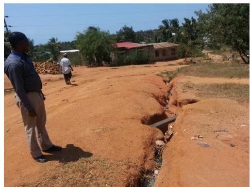
Figure 3: Sign of Soil Erosion along the Proposed site for Water Drain at Chikongola
