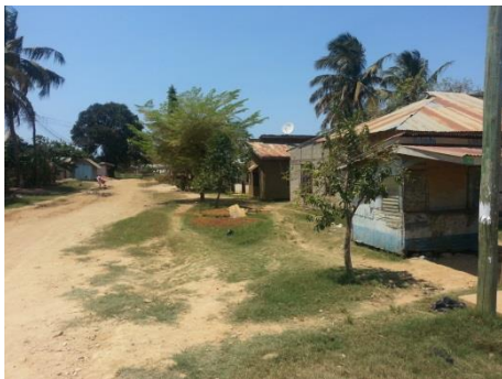
Figure 5: People damaged drainage structure to reduce flooding along Chuno Road
