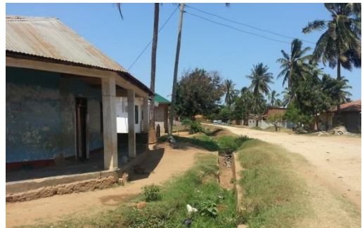
Figure 8: Water Supply pipe near Zambia Road at Likonde
